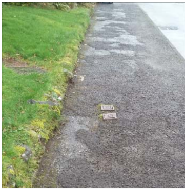
Photo above shows Footway deterioration Nant Drive, Oban. Photo on right shows recently resurfaced footway in Lochside Street , Oban
